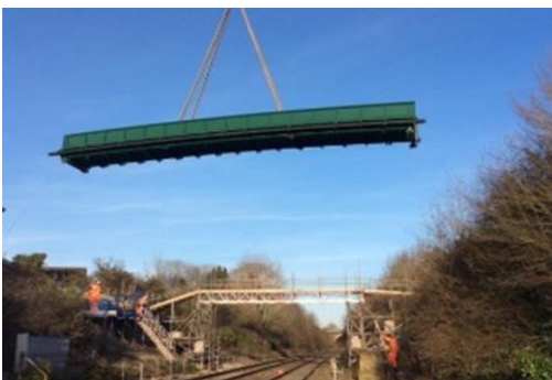
Placing the new bridge into position
