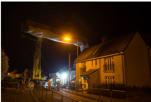
Lifting out the old bridge
